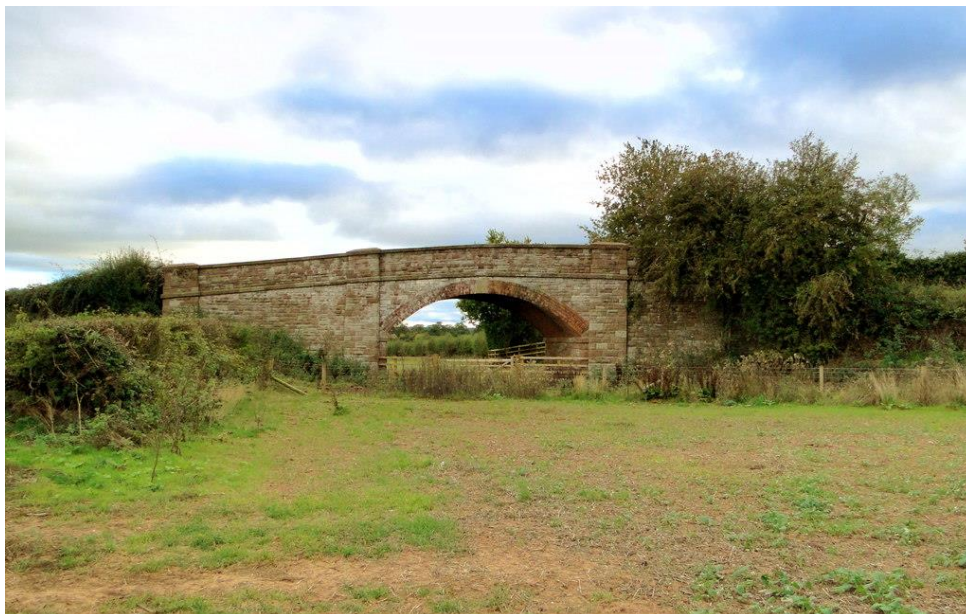
Former railway bridge at Tiller's Green
